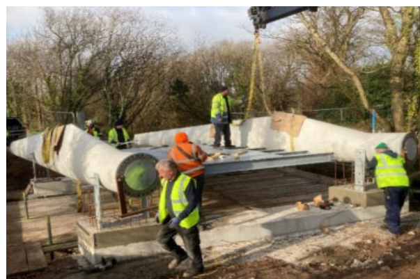
Pedestrian bridge: using 2 8.5 m WTBs as side girders that transfer the loads from a concrete deck to the supports
