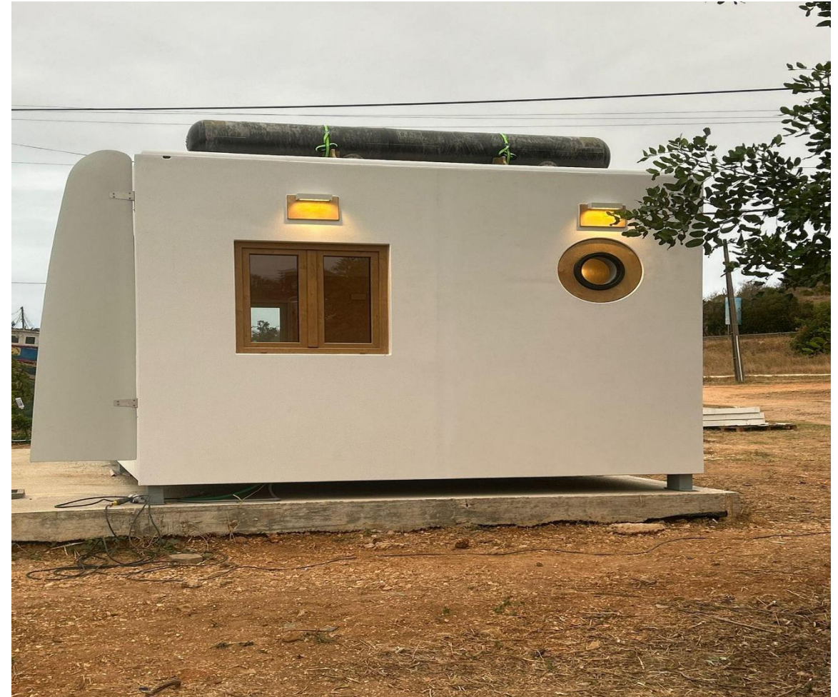
Demonstrator side showing the 3d printed naval window
